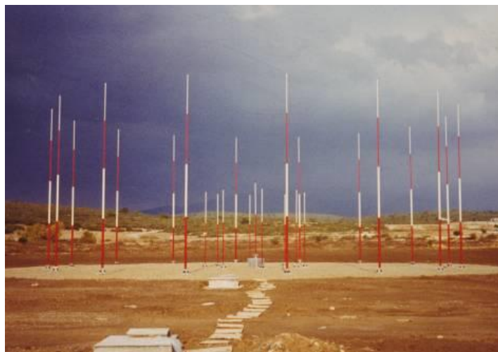
Figure 3: Typical antenna array for strategic HF interception and direction-finding system
